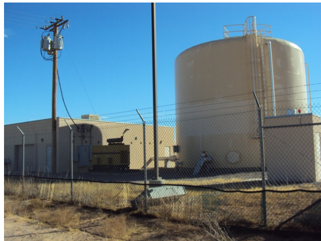
Border Area Tank and Booster Station
