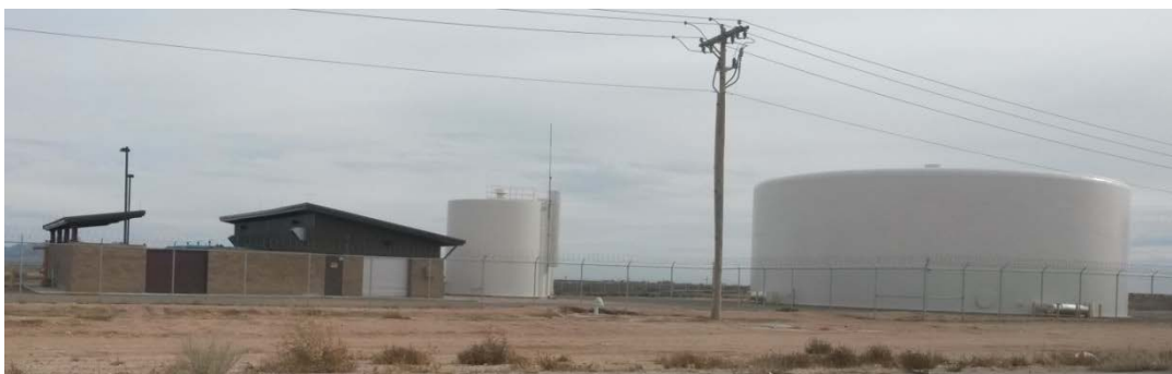
Santa Teresa Industrial Park Arsenic Treatment Facility and 2.0 MG Tank
