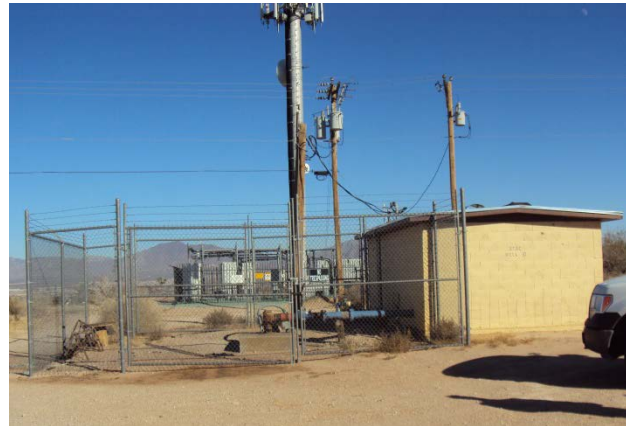
Well 31 in the Santa Teresa Community Service Area
